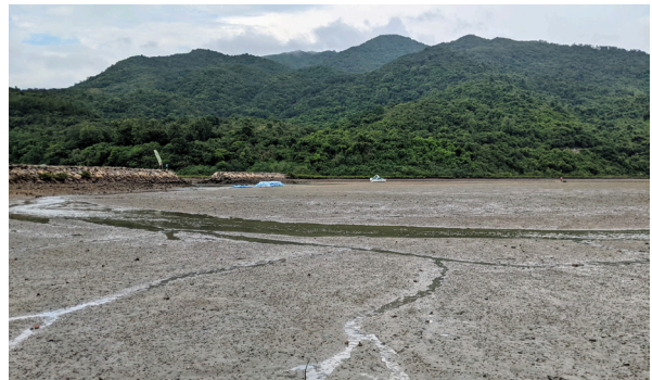
Figure 20. displaying the SK breakwaters from within (KLHLW beach).
