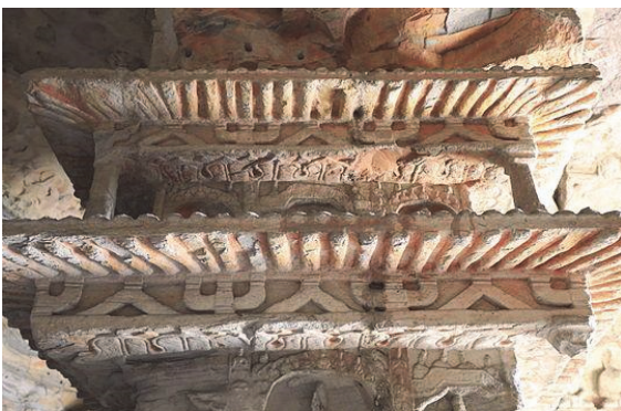
Figure 7. Chinese wooden architectural elements such as Dougong imitated on the pagoda placed at the centre of 2nd grotto in Yungang Grottoes in Northern Wei.
